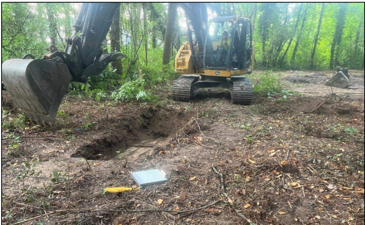
Figure 14. Example of trench excavation, view to the northeast.
