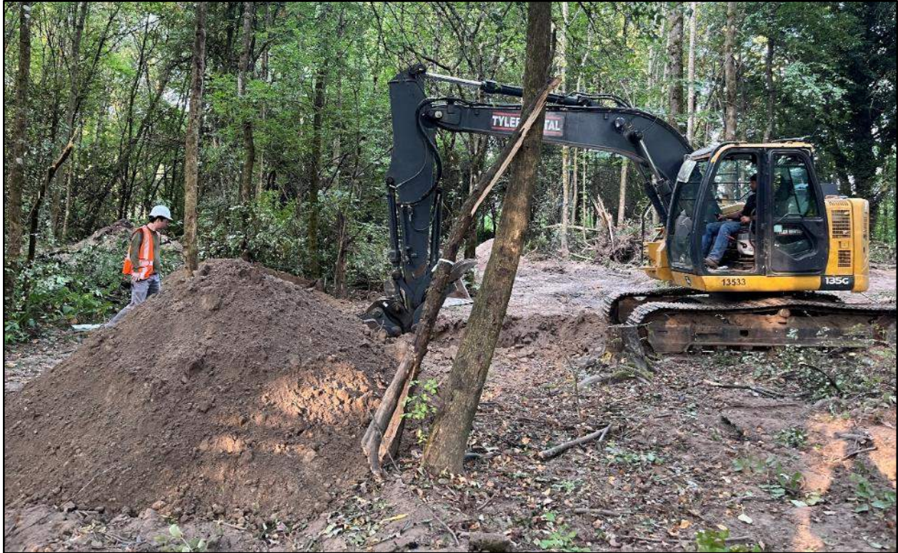
Figure 13. Overview of trench excavation, view to the west.
